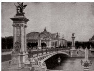
New Alexander bridge, Paris
